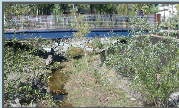
Pedestrian bridge over newly restored Castro Valley Creek
