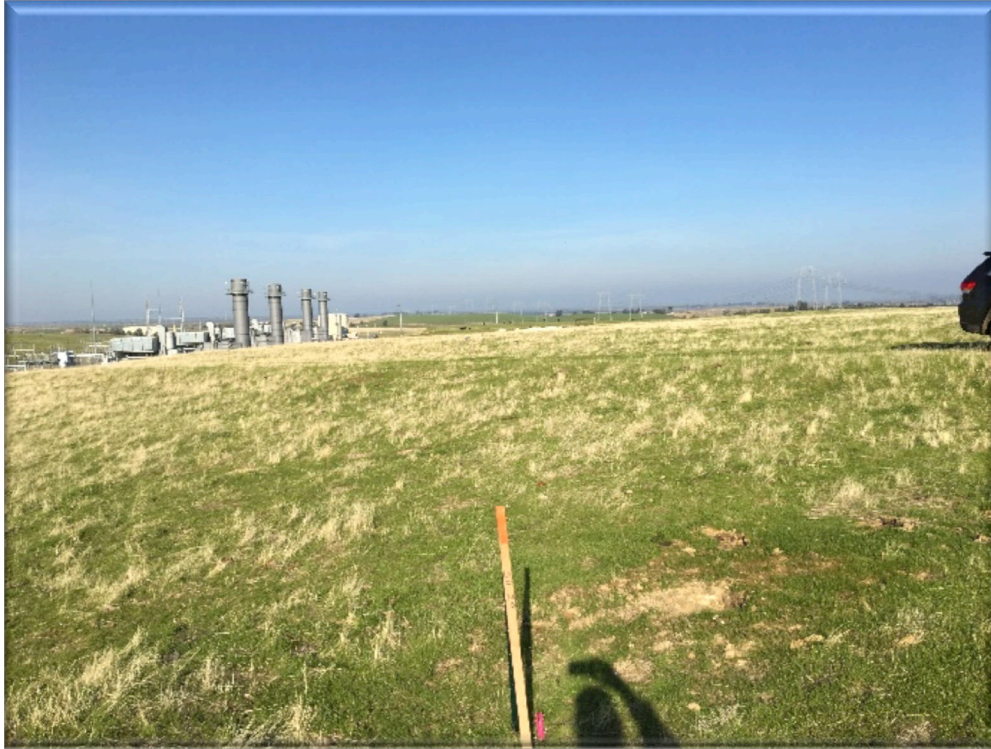
Plate 67. Looking northeast from Site 29B. Moving the turbine an additional 100 feet east across the road onto the flat, open ground and away from the edge of the slope would reduce risk.
